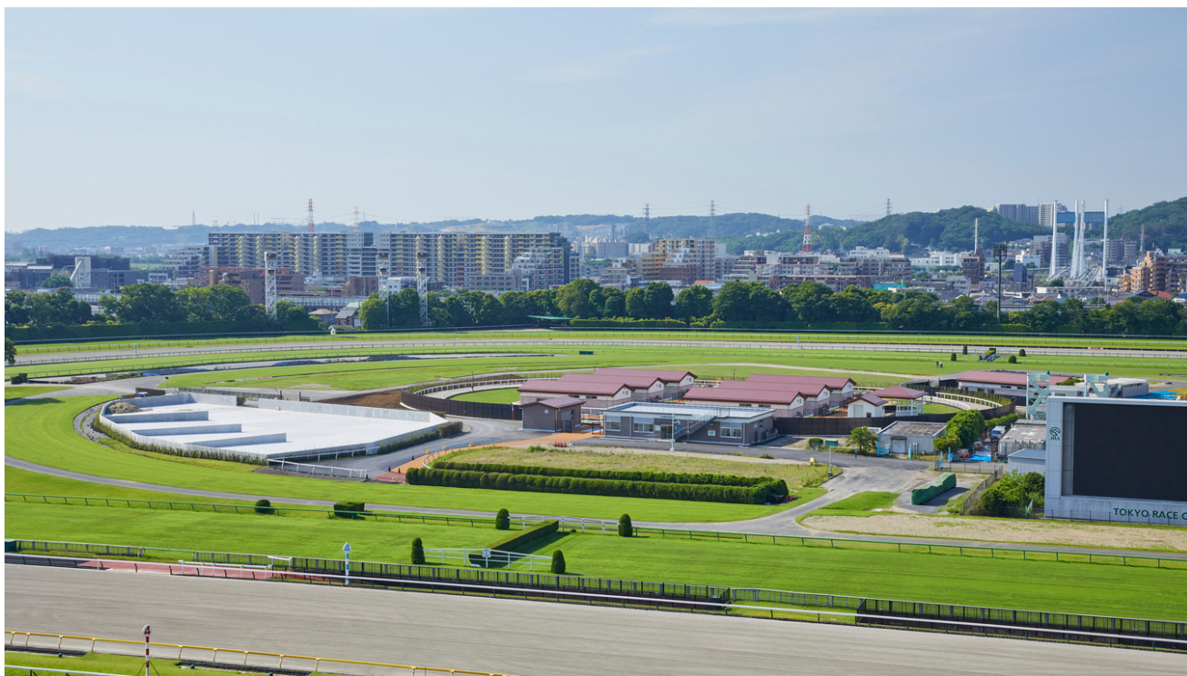
The new international stable at Tokyo Racecourse was designed to make travel and quarantine easier for international competitors
