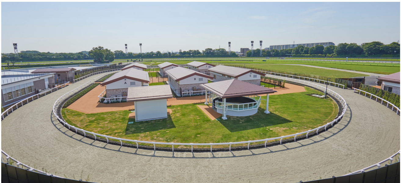
A training track surrounds the new international stable at Tokyo Racecourse
